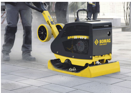
No breakage of paving stones
